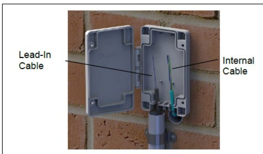
Figure 28. nbn compact NTD with unterminated cables (only white conduit and saddles allowed)
