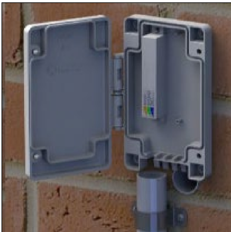
Figure 29. nbn NTD with VDSL2 centralised filter installed (only white conduit and saddles allowed)
