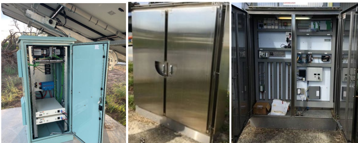
Figure 7. Examples of external rack mount and wall mount customer supplied telecoms cabinet/enclosure
