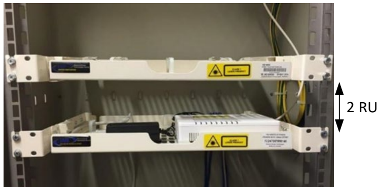
Figure 22. Legacy NTD and PSU variant with 2RU clearance above
