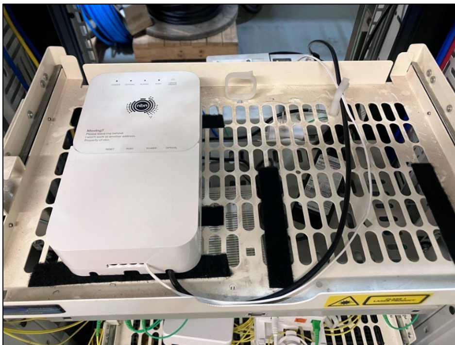
Figure 18. 1-port NTD and rack mount
